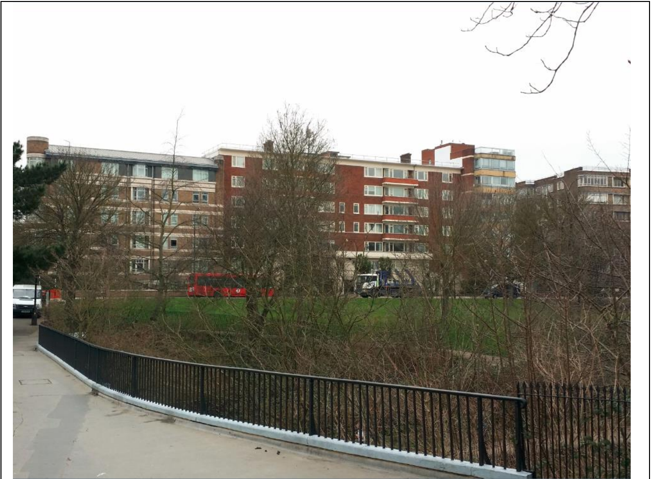
Application site as seen from pedestrian bridge over Regents Canal
